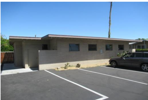
Laundry Room - Exterior
